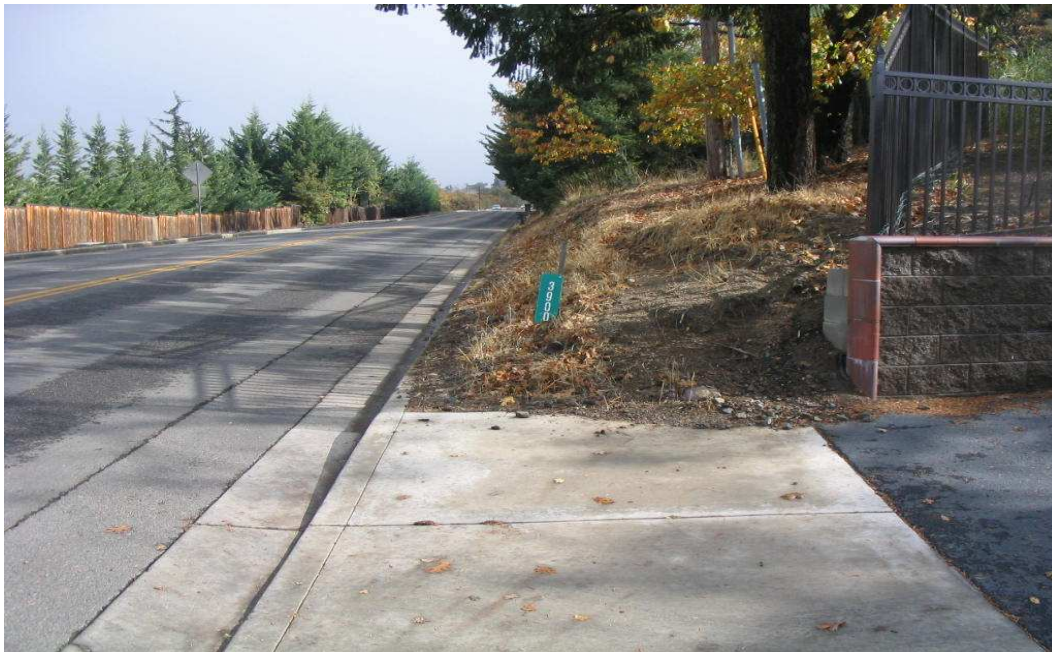
(Above) – Preconstruction photo of the Hillcrest Sidewalk Improvement Project.
