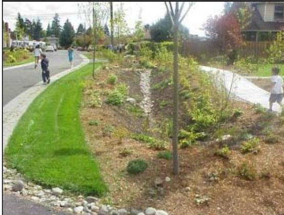
The figure above depicts a street with bioswale along a downgrade edge. The photo shows a built example of a street with a bioswale edge.
